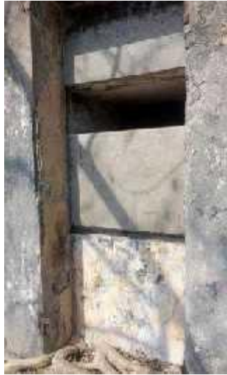
The walls on this casemate are about 1.5 meters thick
