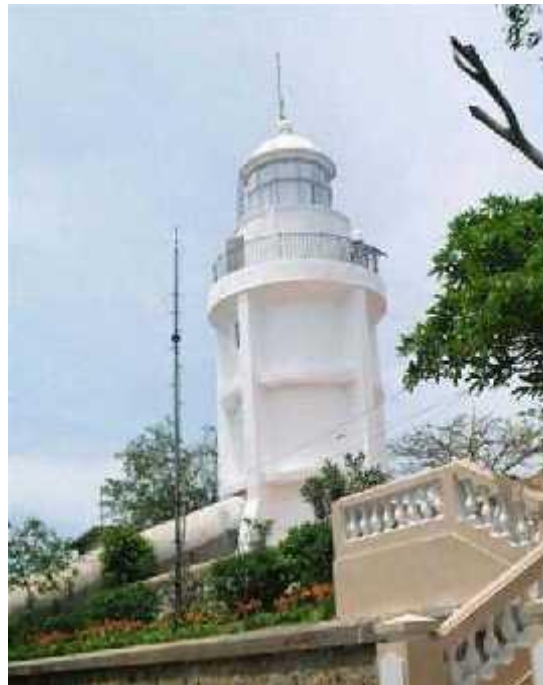
The light of a 1,500-watt lamp in the Yung Tau Lighthouse on top of Nui Nho (small mountain). Boats as far as 56 kilometers offshore can see the two strong beams from the country's oldest lighthouse.
