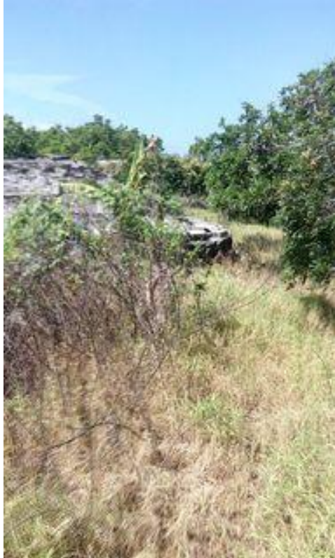
The top of the Bunker
