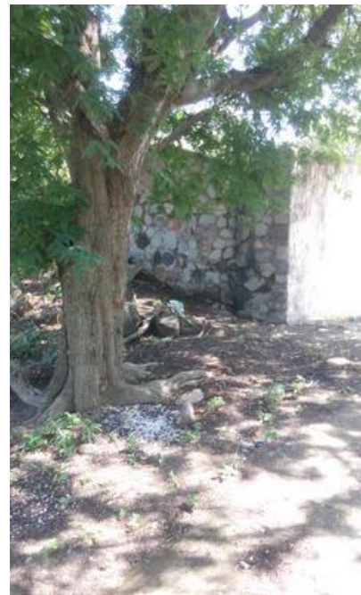
The Left of the Bunker
