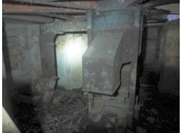
Looking up to where the blower/exhaust connects to the gun turret
