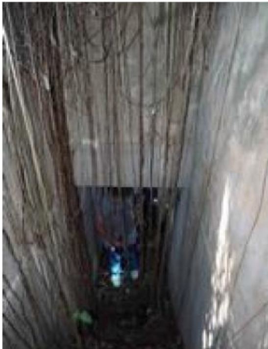
Looking down into Section 4
