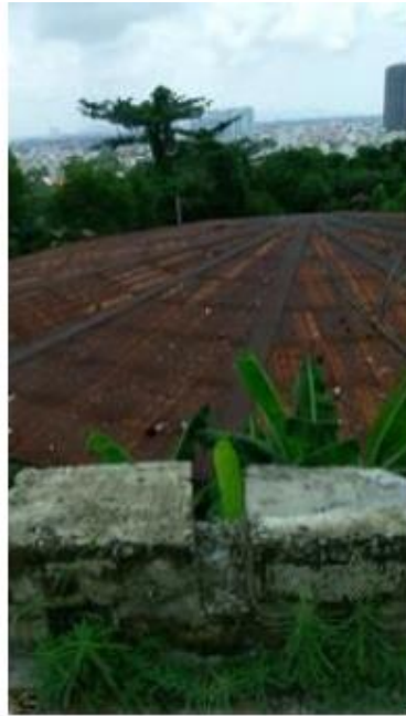
The roof of the tank
