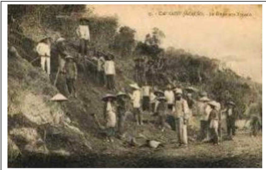
Vietnamese Labourers building the Road to the Light House
