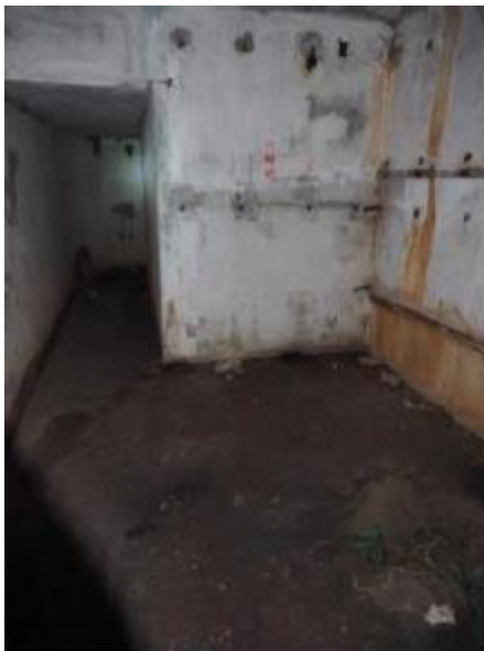
The storage room of Section three .
