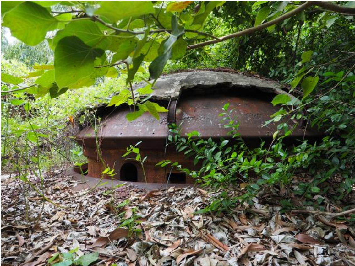
The Gun cupola situated on the roof of the Fort, in it's partially raised position.
