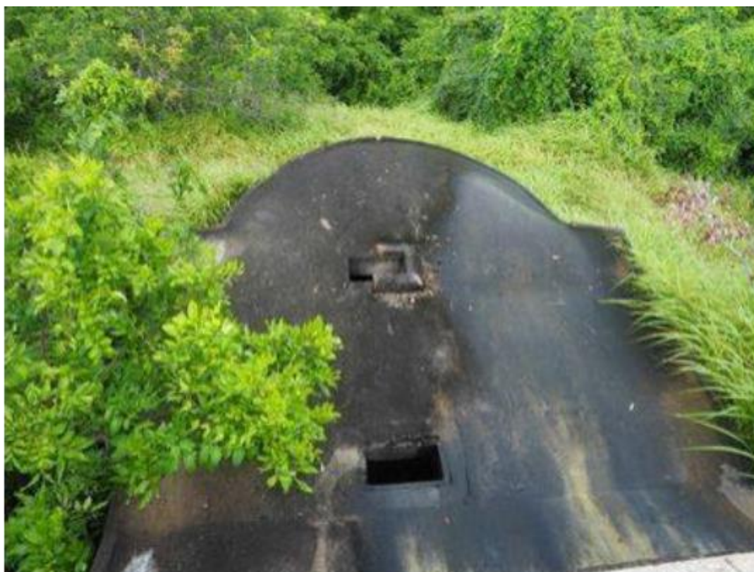
Looking at the top of Section Two .
