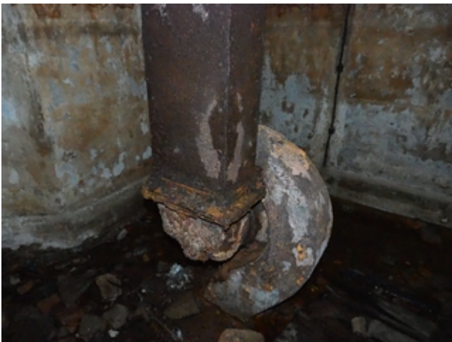
Here is a blower or exhaust fan that is connected to the gun. You can also see the position where the electric motor was placed to drive it.
