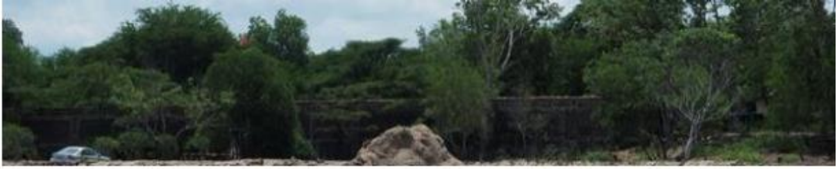
Part of the external wall (right-hand side)
