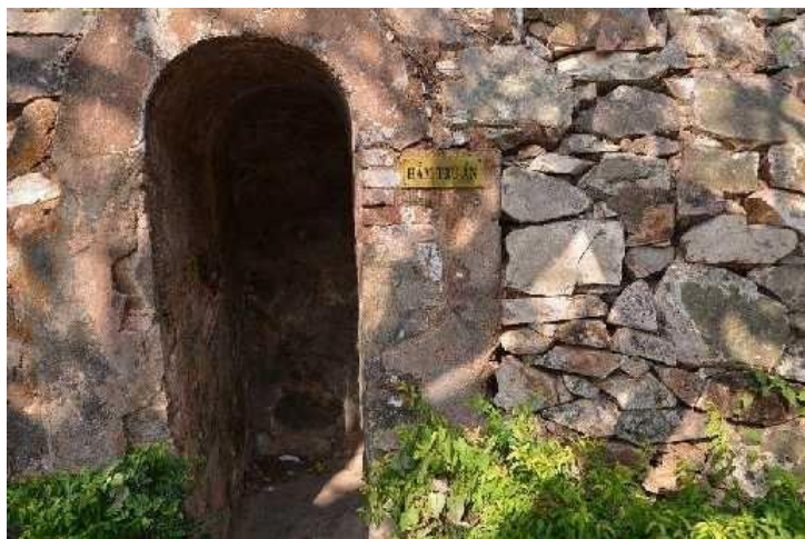
Ham Tru An.....Safety Tunnel ...Shelter
