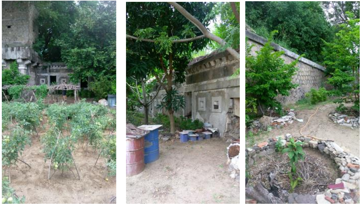
Looking at the right-hand side of the fort which is longer than the left side.
