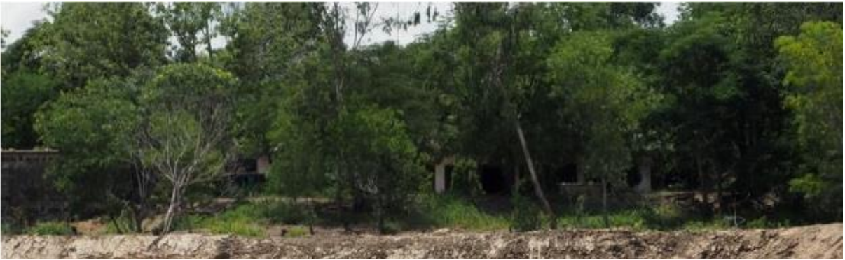
Part of the external wall (left-hand side)
