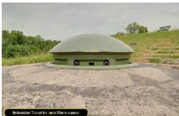
Schneider Turret for twin 75mm canon
