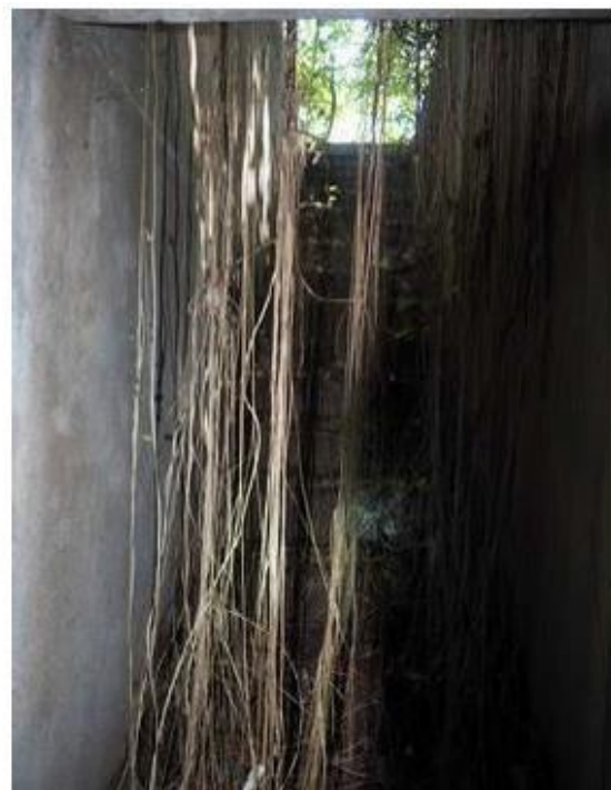
Looking up from Section 4
