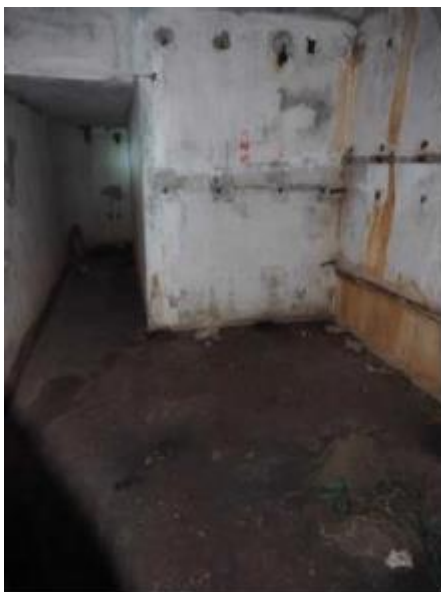
The storage room of Section three.
